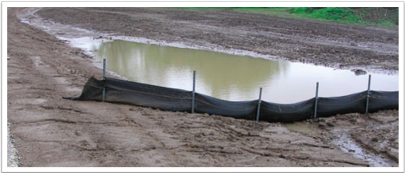
Figure 4-3: Silt Fence
