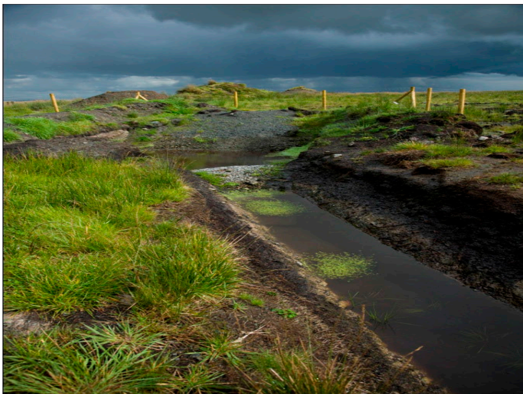
Figure 2-4: Swale draining to Settlement Pond
