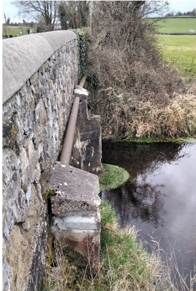
Figure 3-3: Existing Philipstown Bridge Watercourse Crossing at TDR Node No. 29/30
