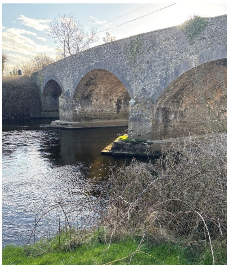
Figure 3-2: Existing bridge on BARROW_090 River
